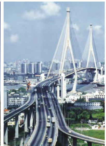
建设银行支持建设的上海杨浦大桥 The Yangpu Bridge in Shanghai, built with the support of CCB.
